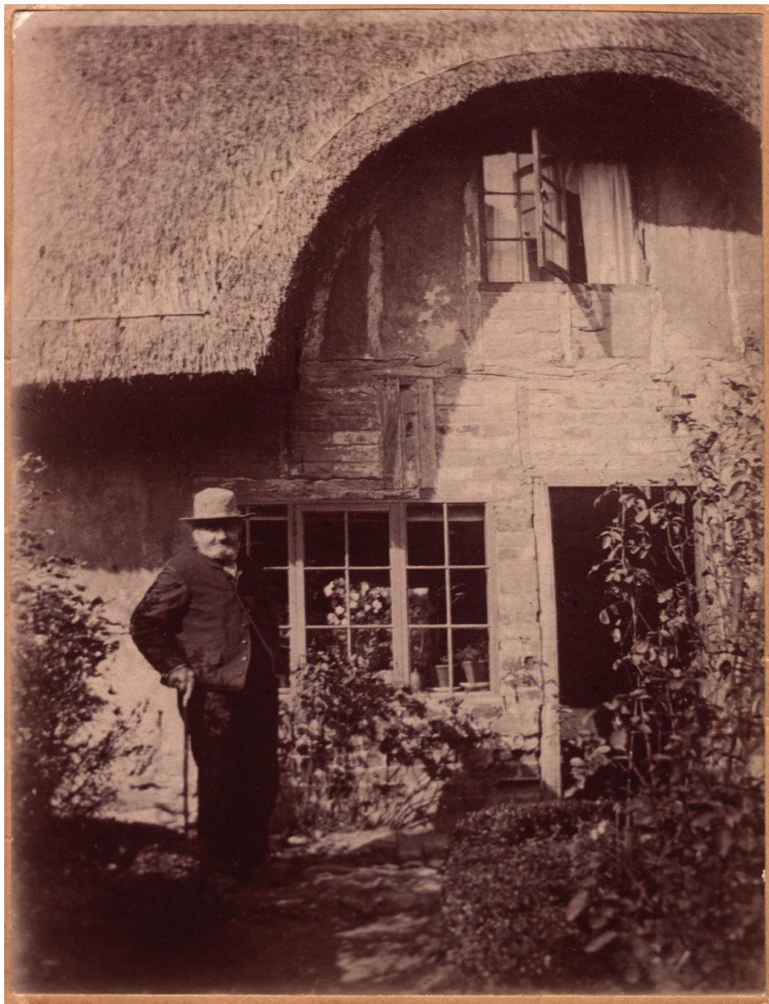
Cottage at 20 Church Street prior to demolition and building of current property. From the Village Old Photo Collection.... Courtesy of Mr. Eric Furr.
